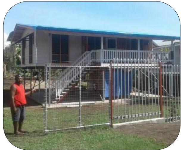
KOKOPO: Christine’s husband, Kenneth Kamit in front of their recently built house at Kinabot
